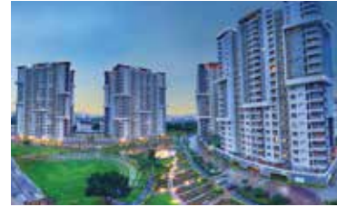
GREENAGE Hosur Main Road, Bengaluru
