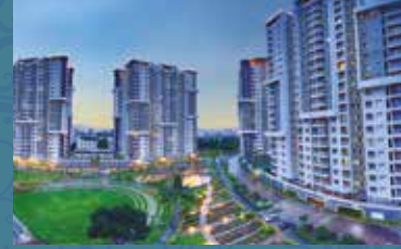
GREENAGE Hosur Main Road, Bengaluru
