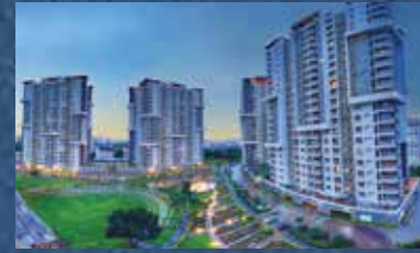
GREENAGE Hosur Main Road, Bengaluru
