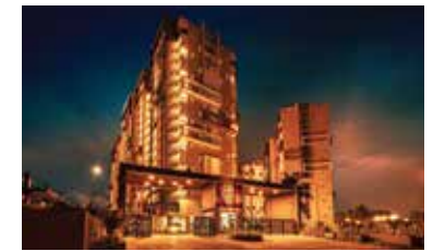
East Crest Near Budigere Cross, Bengaluru
